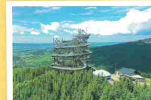
SKY BRIDGE & SKY WALK IN DOLNÍ MORAVA
